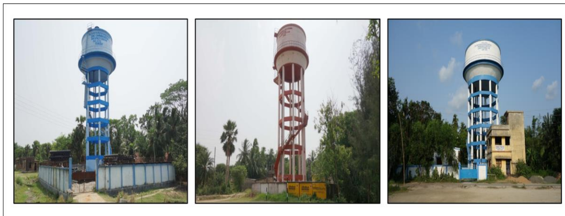
Figure 2(b) Overhead reservoirs to distribute treated surface water to thousands of households via piped-networks. Administrative names, from left to right: Diamond Harbour I (Zone–2), Diamond Harbour II (Zone–6), Uttar Raipur Budge Budge I
