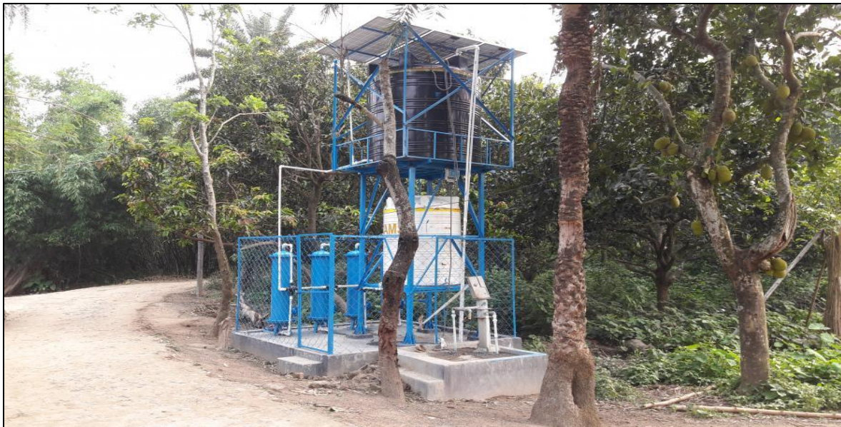
Figure 8 A typical ARU located in the Tajpur habitation of Uttar Tajpur village under Karimpur-I block (GP Pipul Baria) in district Nadia
