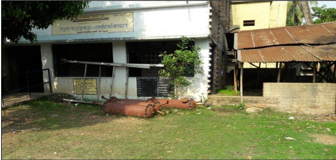
Figure 12(a) Discarded exhausted media of an ARU of Asarpara habitation of Bagula village under Hanskhali block (GP Bagula-I) in district Nadia
