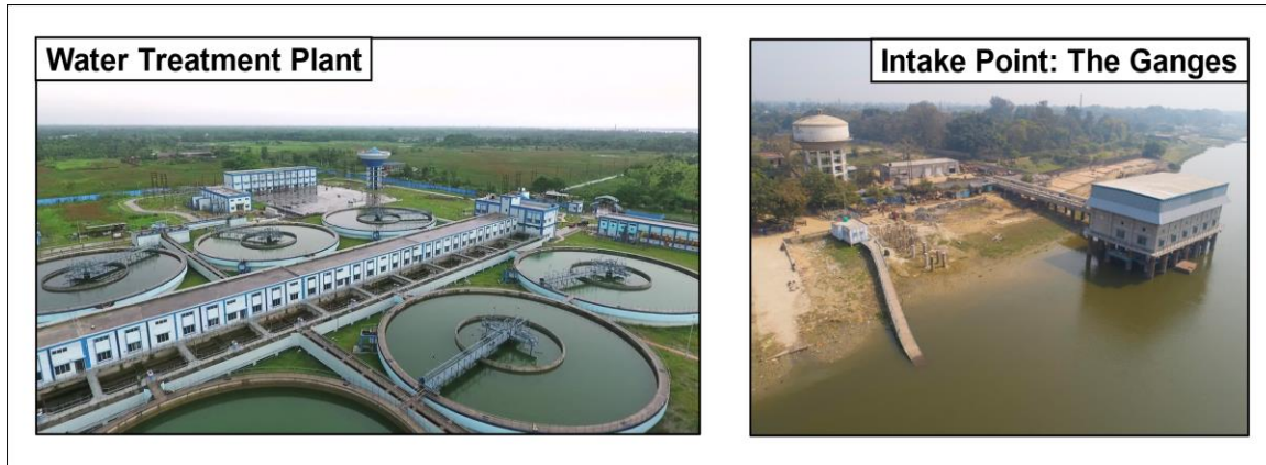
Figure 2(a) Treatment plant of a mega surface water-based water-supply scheme (Falta–Mathurapur) in district South 24 Parganas, West Bengal. Arsenic-free surface water of the perennial river Ganges is abstracted for Piped–Water–Supply Schemes (PWS)
