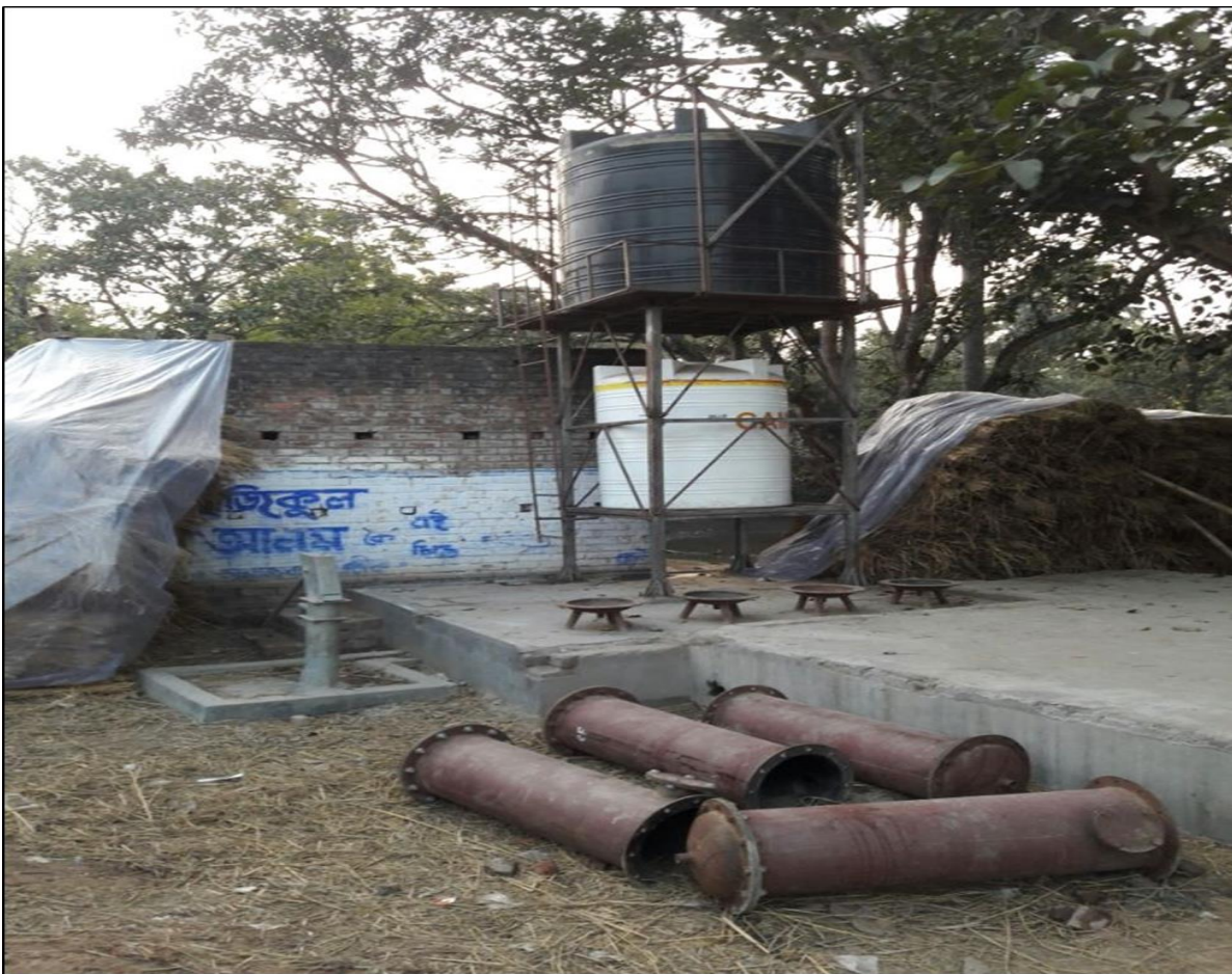
Figure 12(b) Discarded exhausted media of an ARU of Mahatpur habitation of the Mahatpur village under Bhagawangola-I block (GP Sudarpur) in district Murshidabad
