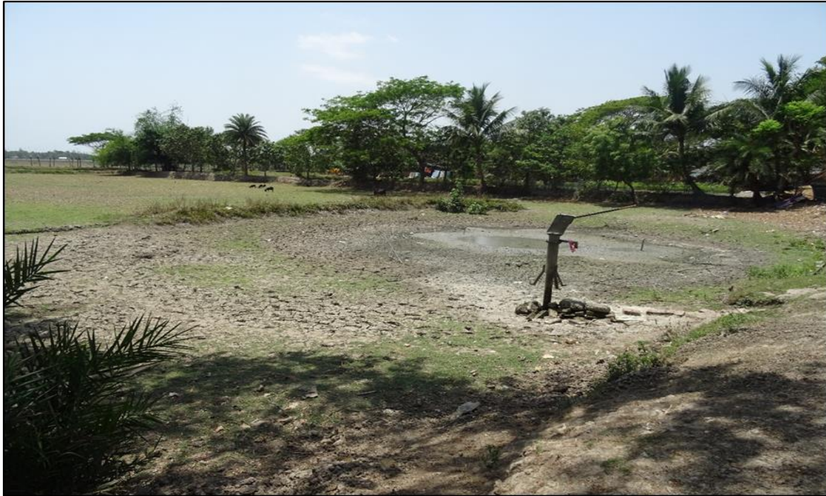
Figure 4 A typical hand-pump-fitted tubewell in rural West Bengal, that has now been abandoned after detection of arsenic in groundwater
